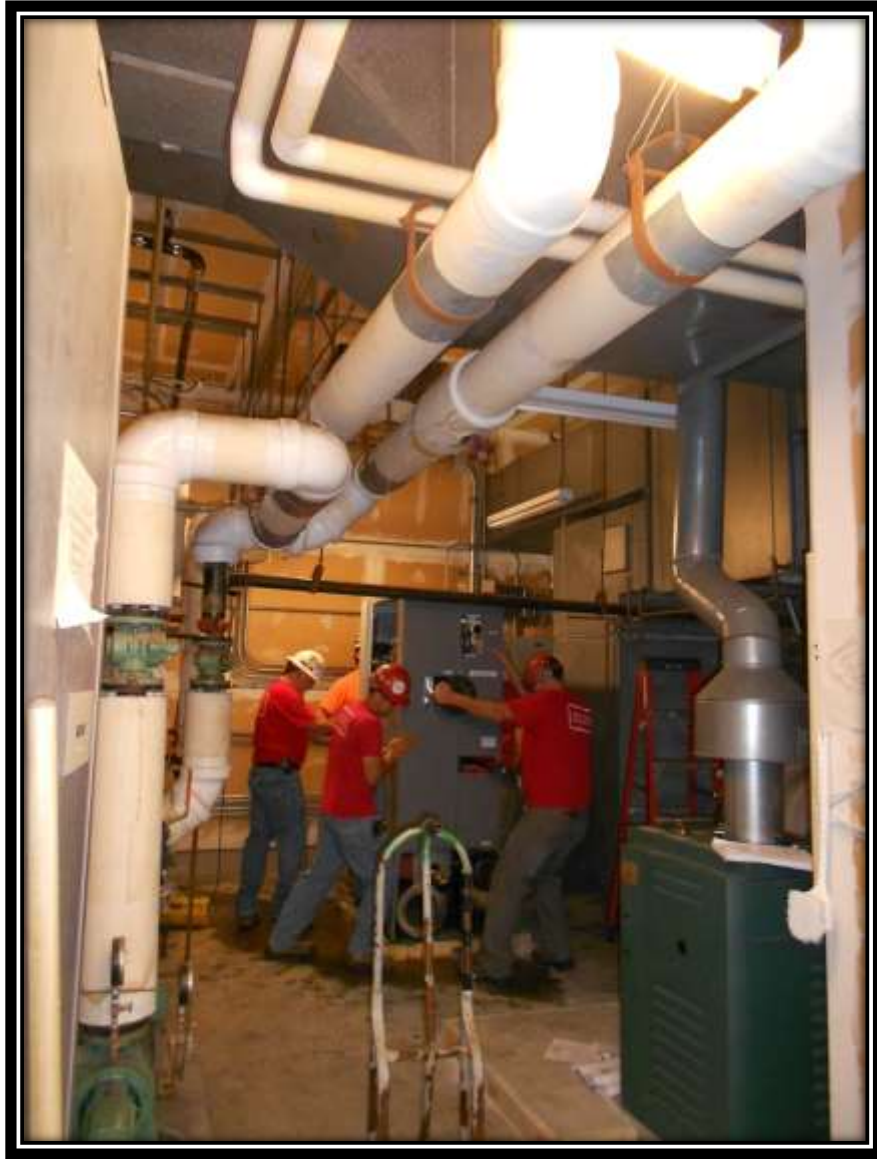
Installing new Boiler #1 unit
