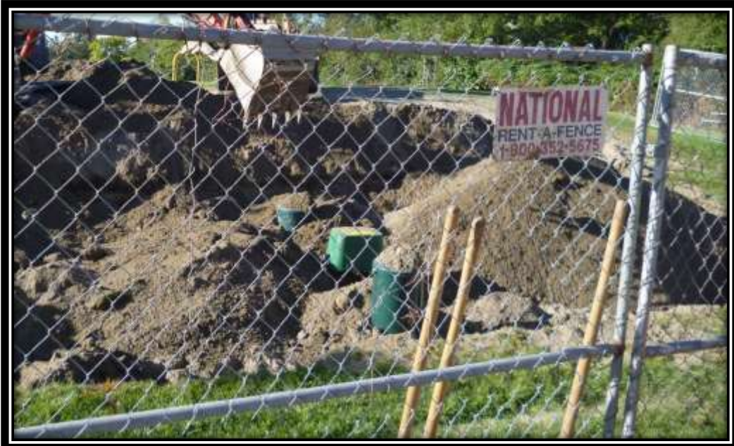
Earthwork construction for installation of underground propane tank
