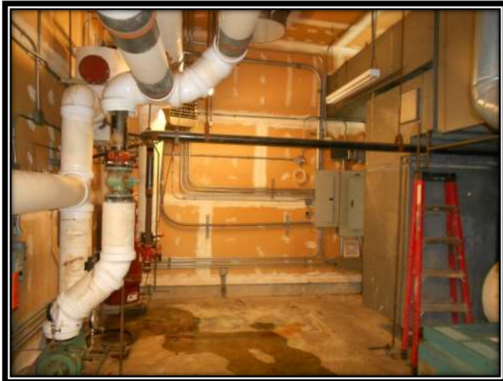
Location of existing Boiler #1 following demolition
