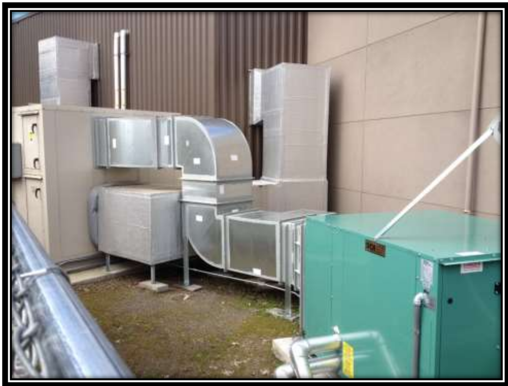
Completing the finishing touches prior to equipment start-up
