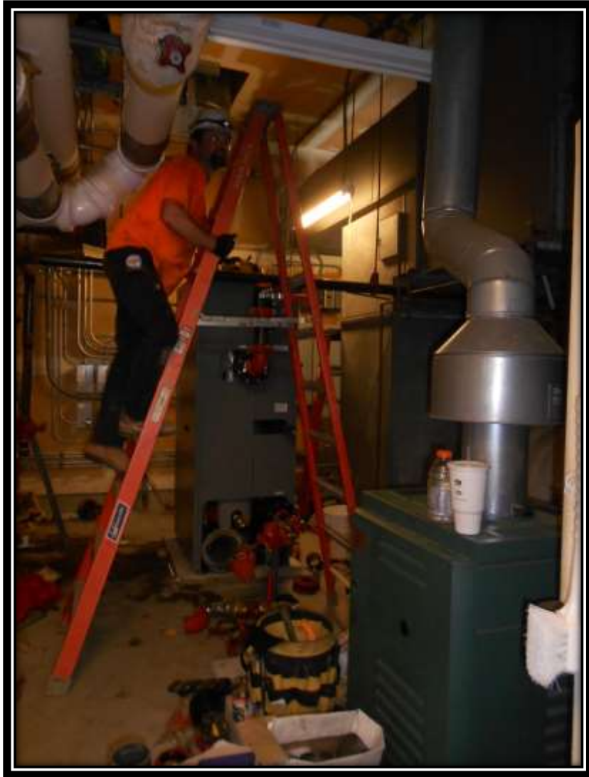
Work in progress View of new Boiler #1 after final placement
