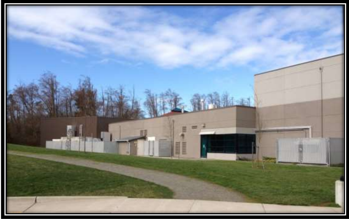
Back of building after construction
