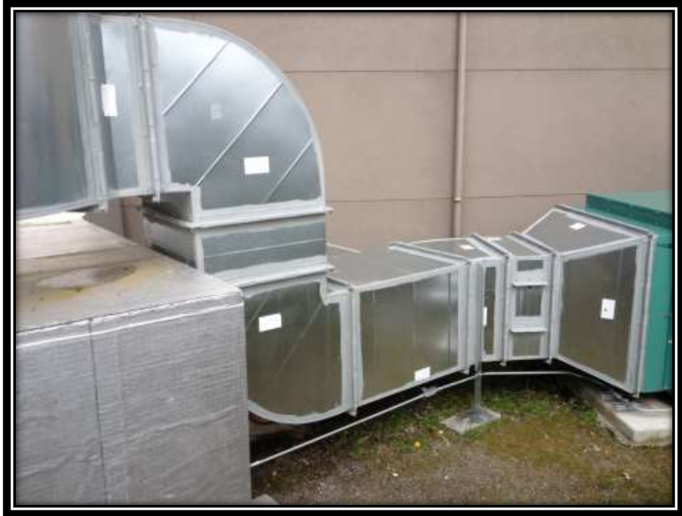
Installing remaining ductwork on outdoor unit
