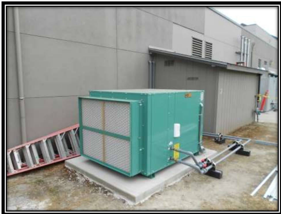
Placement of new outdoor unit following pad completion
