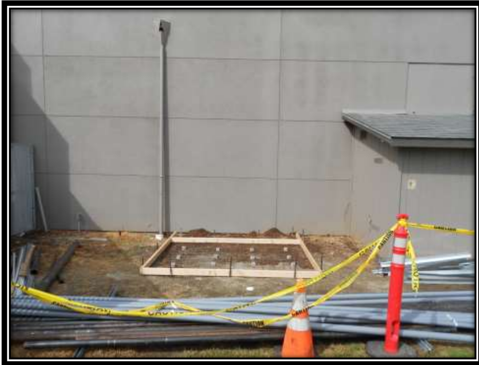
Prepping to pour concrete pad for outdoor unit placement
