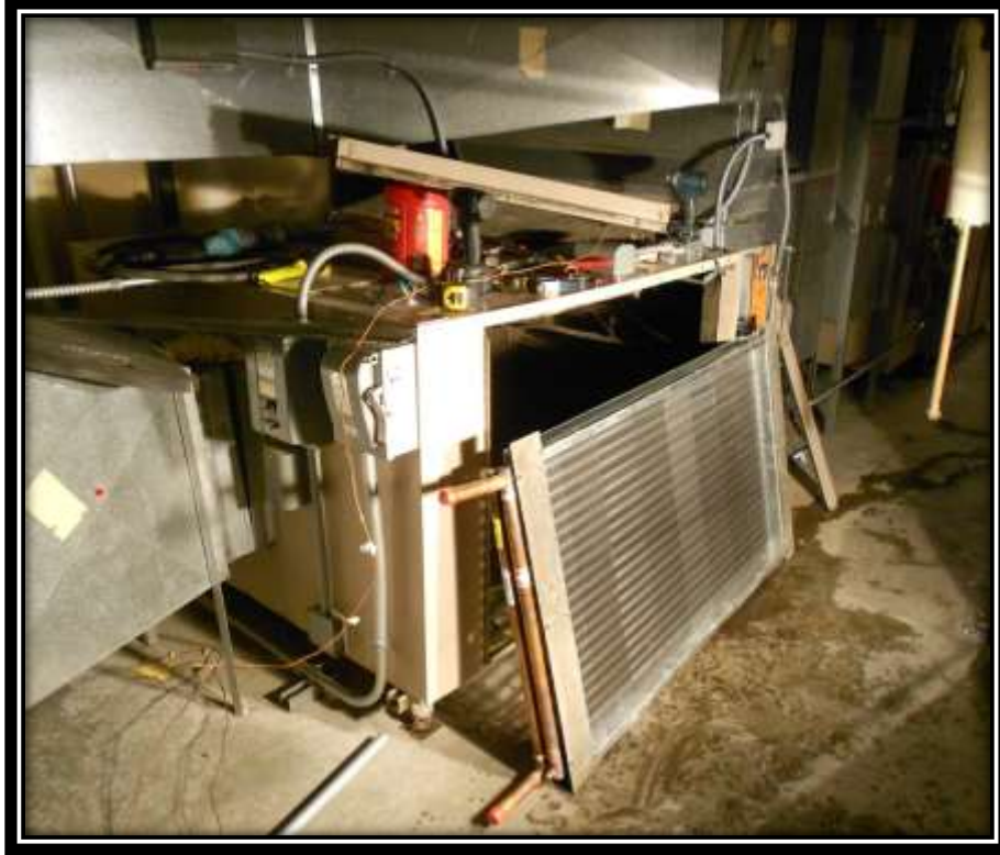
Coil installation in progress
