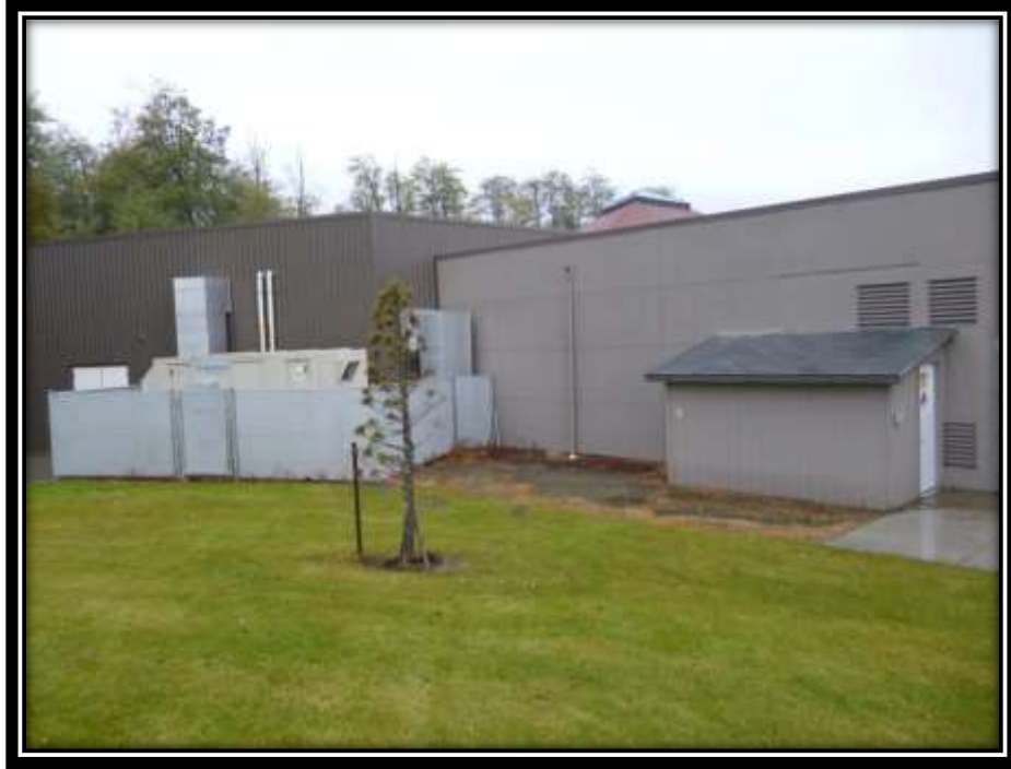
Back of building prior to construction
