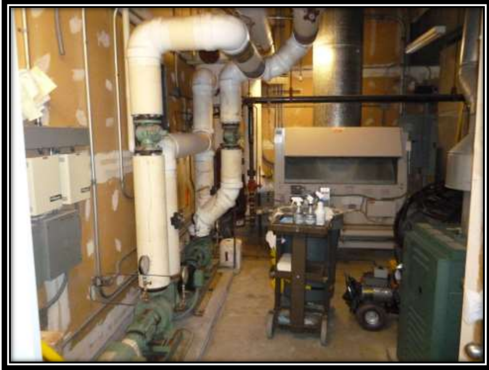
Existing Boiler #1 prior to removal and replacement
