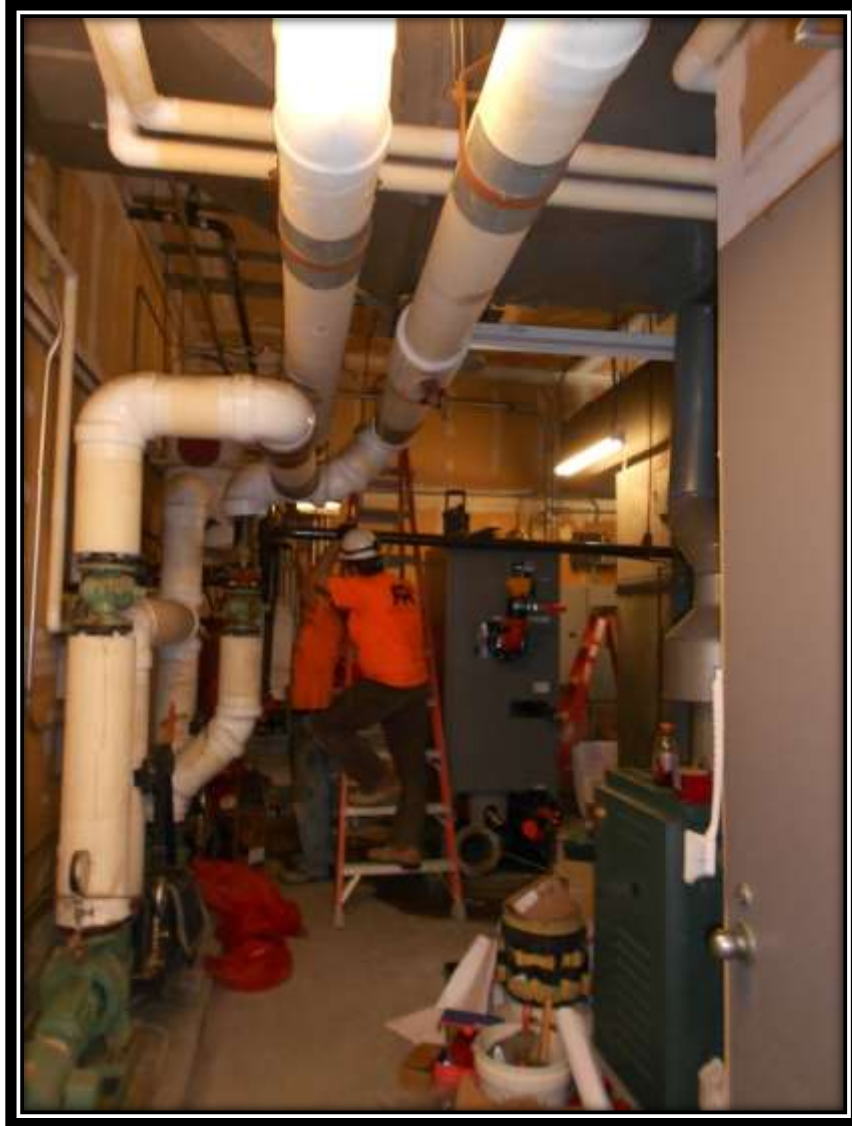
Boiler piping activity in progress
